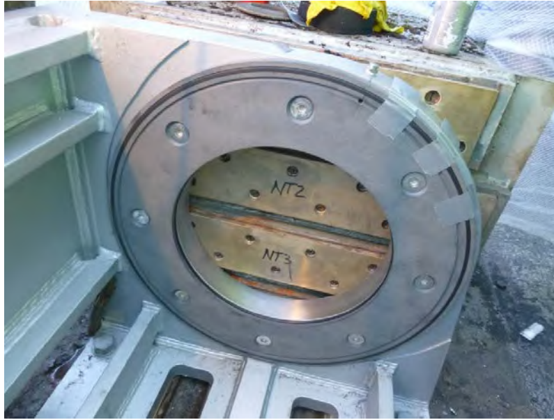
Figure 12-26. Spillway Tainter Gate Trunnion Thrust Washer.
