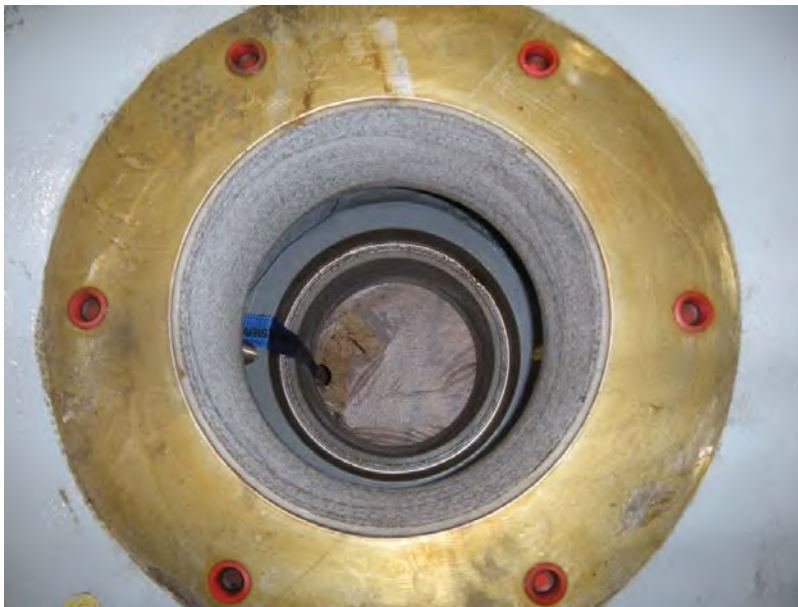
Figure 12-32. Wicket Gate Operating Mechanism Bushings.
