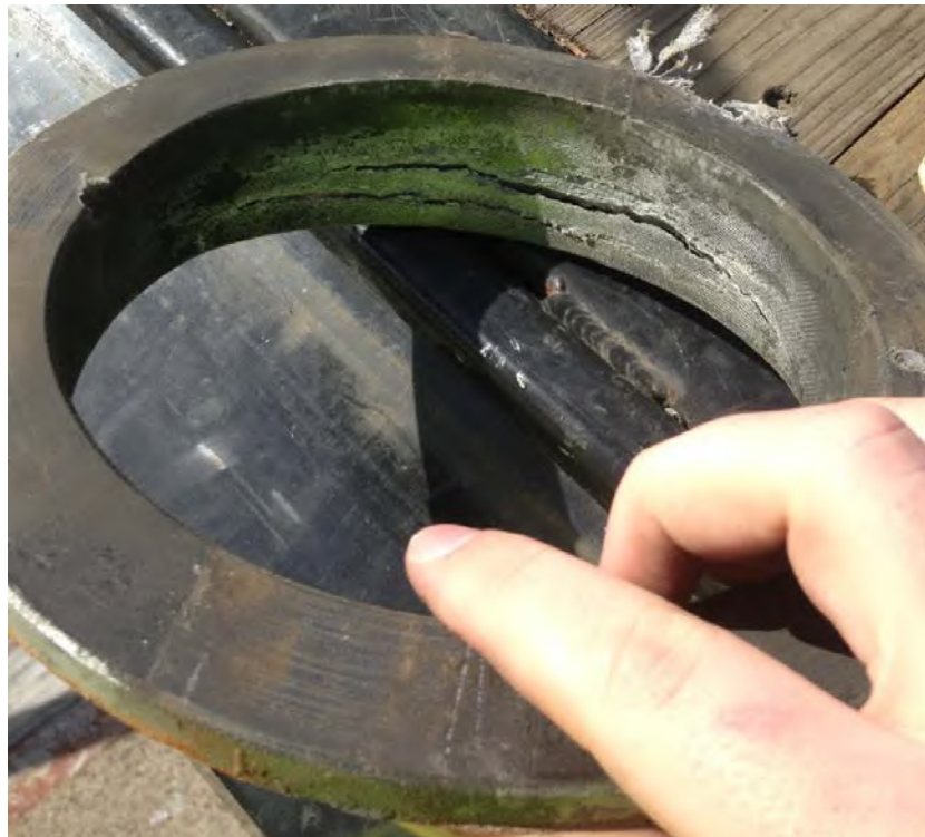
Figure 12-16. Crushing Failure of Textile-Reinforced Composite Self-Lubricated Component.
