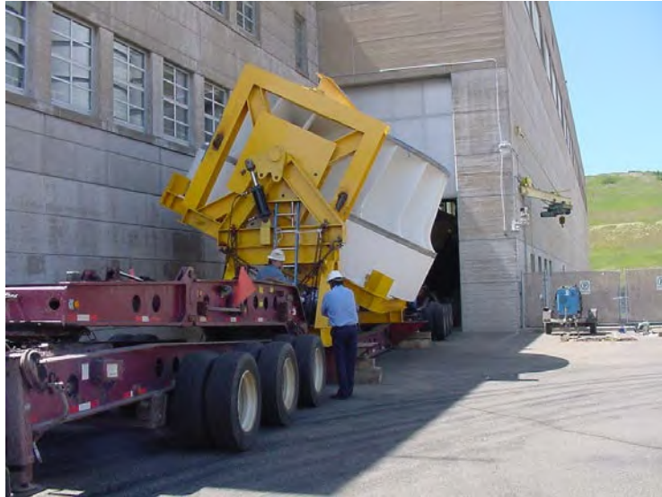
Figure 9-6. Francis Turbine Runner Transported into Powerhouse.
