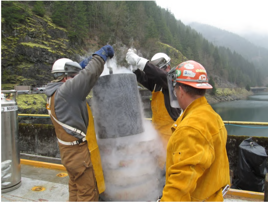
Figure 12-24. Spillway Tainter Gate Trunnion Bushing Freeze Fitting.
