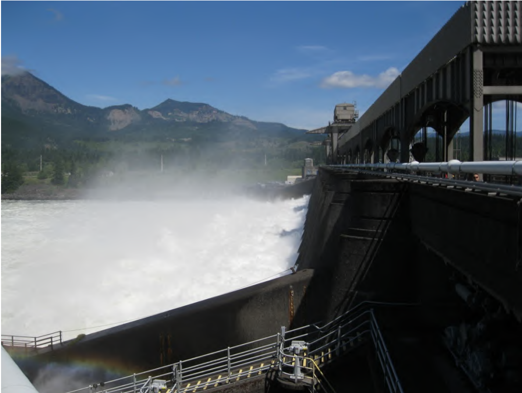
Figure 13-1. Bonneville Dam Spillway on Columbia River.
