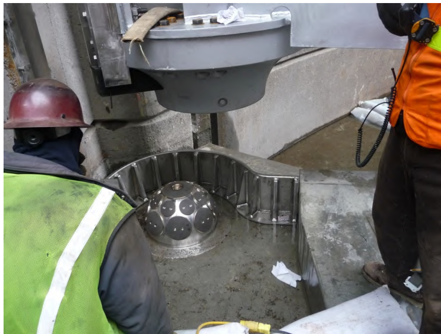
Figure 12-21. The Dalles Dam Miter Gate Pintle Installed.
