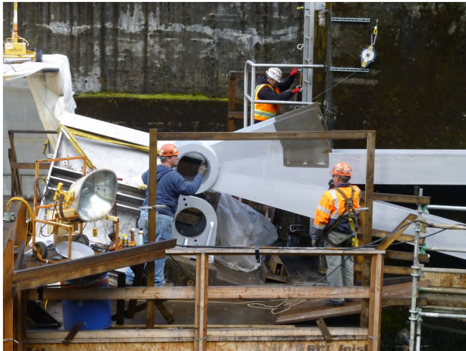
Figure 12-25. Spillway Tainter Gate Trunnion Bushings.
