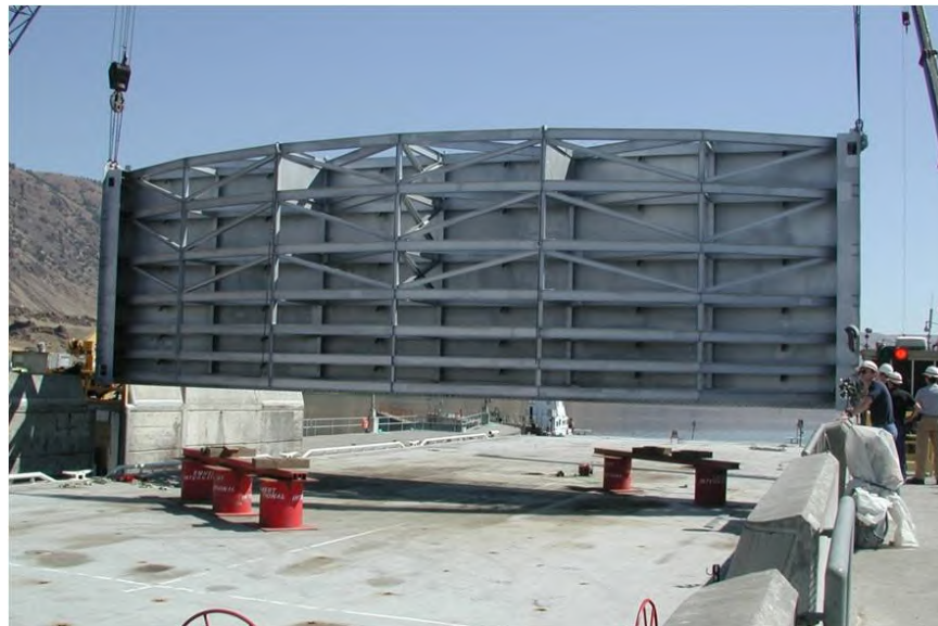
Figure 12-28. John Day Dam Vertical Lift Gate.
