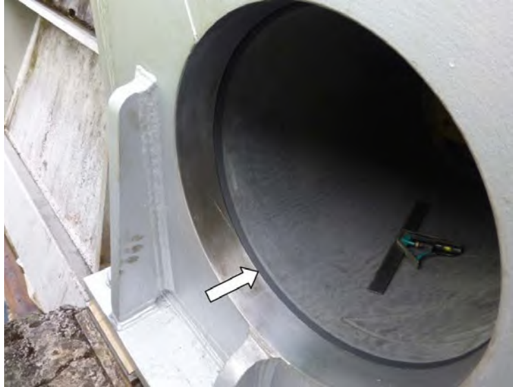
Figure 12-18. PTFE Spring-Loaded Deflection Seal (Indicated by Arrow).
